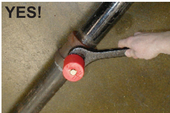
Figure 1: Correct use of designated installation wrench with ESFR Pendent K14 Sprinkler SIN VK500 and sprinkler cap
