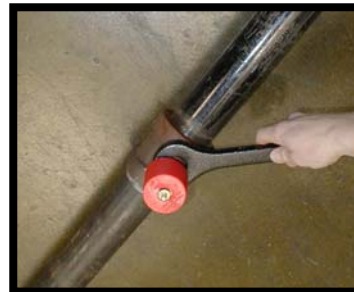
CORRECT (piping is in place at the ceiling)
