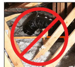
INCORRECT (Exposed piping)
