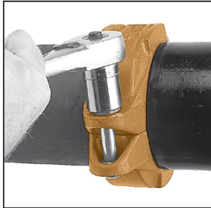
**5 TIGHTEN NUTS**— Tighten the nuts alternately and equally to the specified bolt torque. The housing bolt pads must make metal-to-metal contact.
