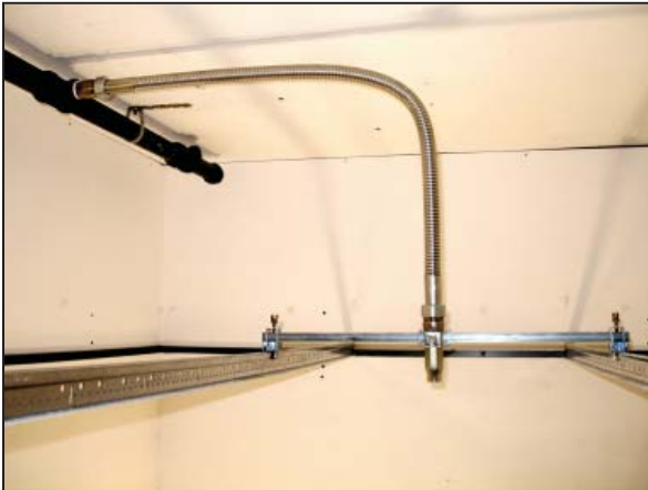
Figure 1: Flexible Sprinkler Drop Installed
