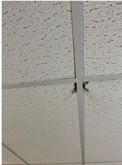
Figure 6: Permanent Damage Observed on Tiles Directly Below the Nozzle Above the Ceiling
