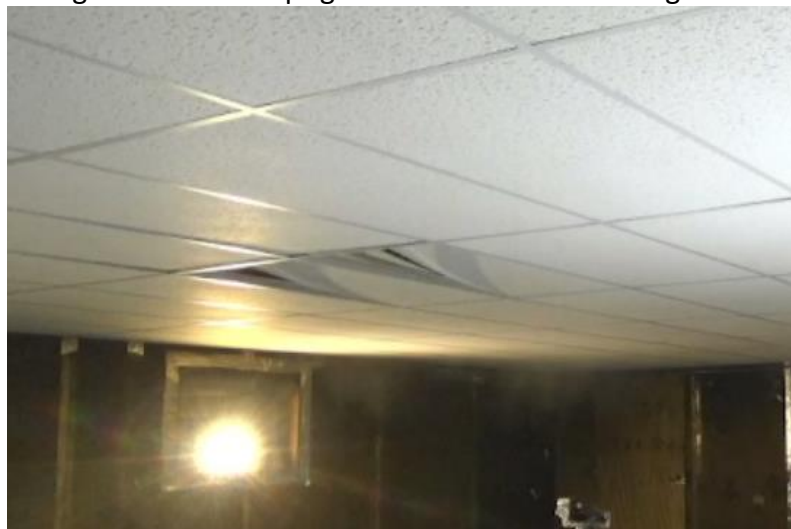
Figure 5: Ceiling Tiles Being Lifted from Grates During System Discharge
