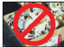
INCORRECT (Protective caps not in place)
