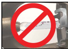
INCORRECT (bulb cracked, fluid missing)
