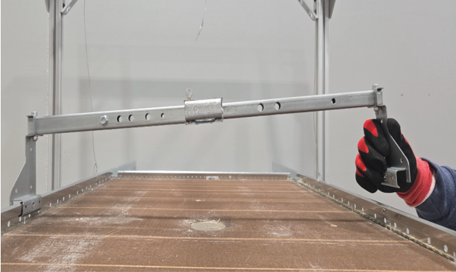
Figure – 1: Apply Pressure on Bracket Legs
