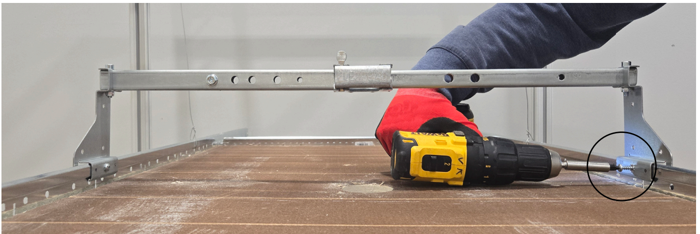
Figure – 2: Install Mounting Screws into T-Bar
