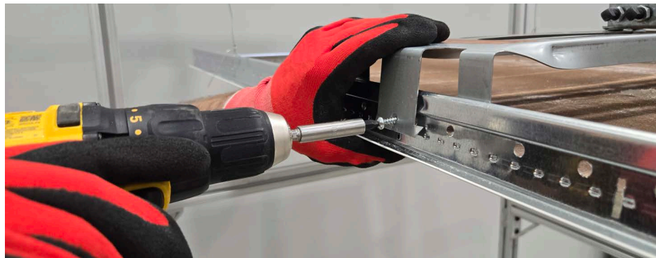
Figure – 2: Fasten Bracket onto T-Bar
