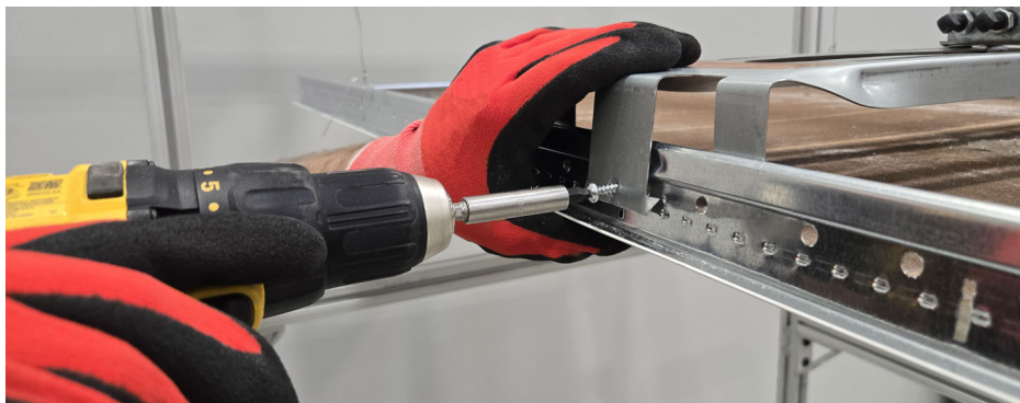
Figure – 2: Fasten Bracket onto T-Bar
