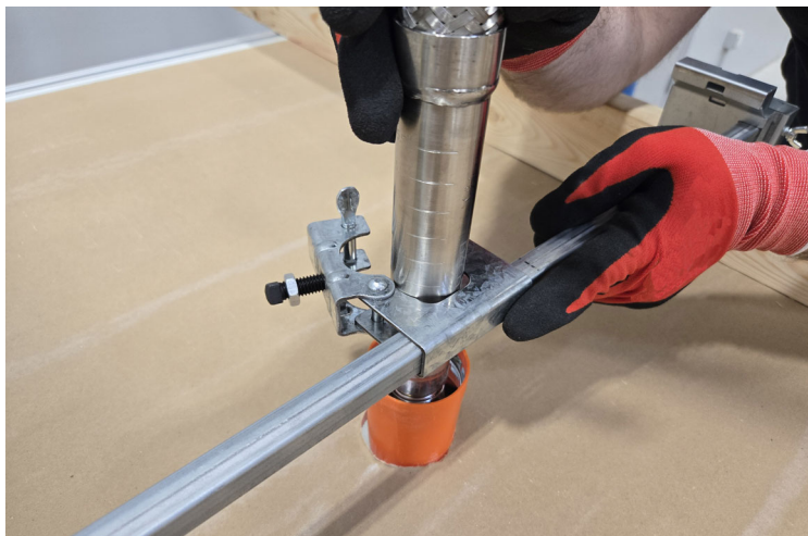
Figure – 2: Place Flexible Sprinkler Hose Assembly into Hub
