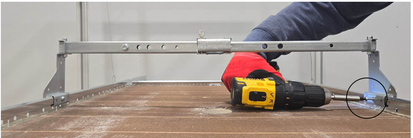
Figure – 2: Install Mounting Screws into T-Bar
