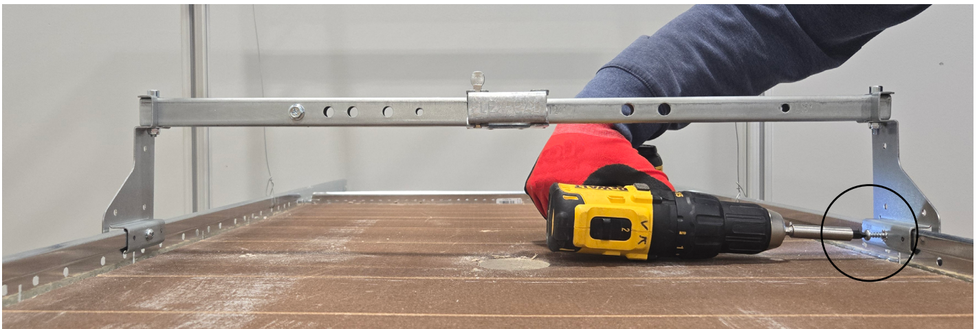
Figure – 2: Install Mounting Screws into T-Bar
