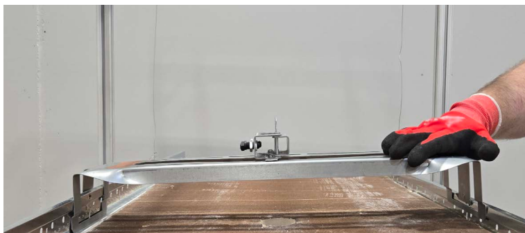
Figure – 1: Downward Pressure on Bracket Leg
