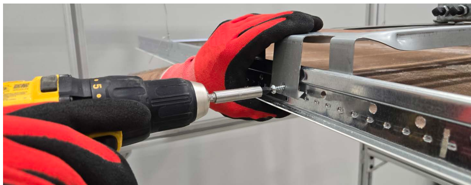
Figure – 2: Fasten Bracket onto T-Bar
