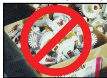
INCORRECT (Protective caps not in place)
