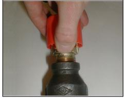
Figure 3: Sprinkler cap being removed from and upright sprinkler.
