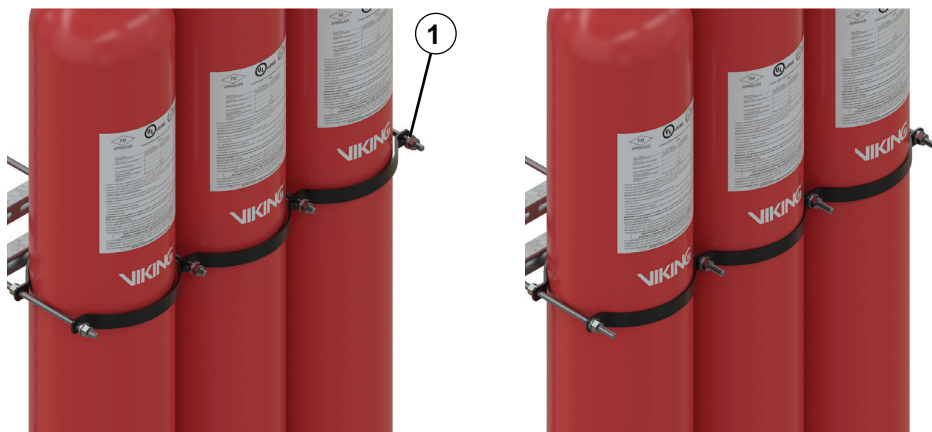
Figure 6.7: Tighten brackets
