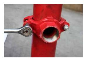
Alternatively and evenly tighten the nuts to the specified bolt torque given below
