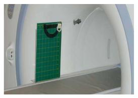
*Figure 3. Sprinkler with large deflection angle. This may pose a hazard in the MR environment.*
