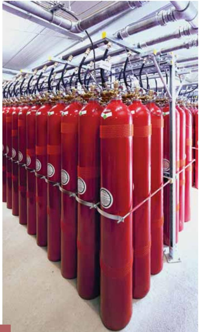
Through the use of Oxexo extinguishing systems, a smaller space for the extinguishing agent supply can be planned in new buildings, which will lower construction costs. In existing buildings, on the other hand, the use of an inert gas extinguishing system often only becomes possible at all thanks to the space-optimized inert gas storage.
