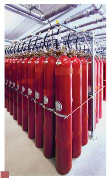
Through the use of Oxeo extinguishing systems, a smaller space for the extinguishing agent supply can be planned in new buildings, which will lower construction costs. In existing buildings, on the other hand, the use of an inert gas extinguishing system often only becomes possible at all thanks to the space-optimized inert gas storage.
